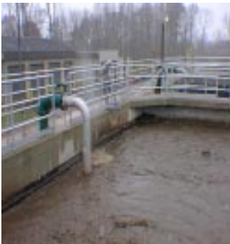
Poor operation of aerobic digesters may result in high P loadings being recycled to the SBRs.
