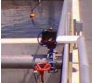
Air control valves should be properly designed and installed to avoid freezing.
